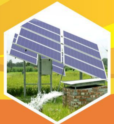
Solar Water Pump
